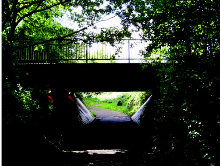
Plate 9 – Typical underpass under Far Moor Lane
